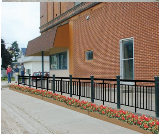
Top: Existing Syndicate Block building.
